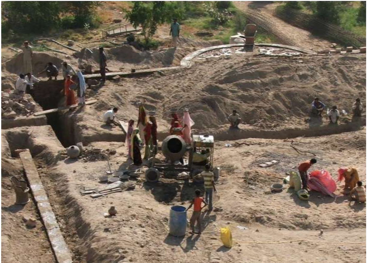
Construction site in Rajasthan
